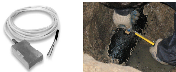
Fig. 6. Superficial temperature sensor and the method of its installation
